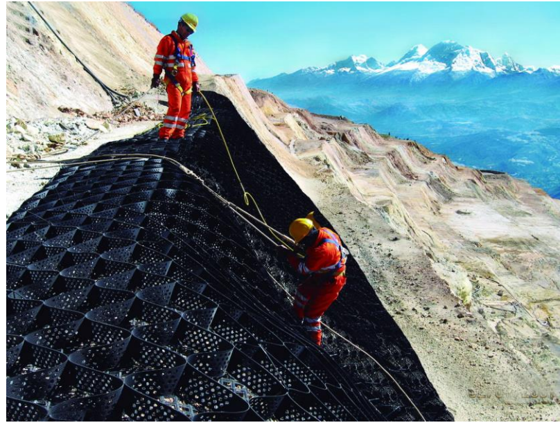
Geocell slope restoration project
