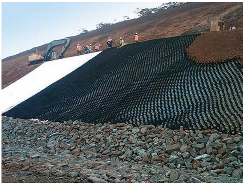
Geocell slope restoration project
