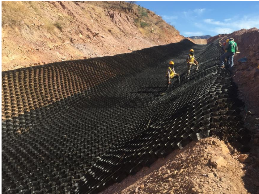
Geocell storm water channel construction
