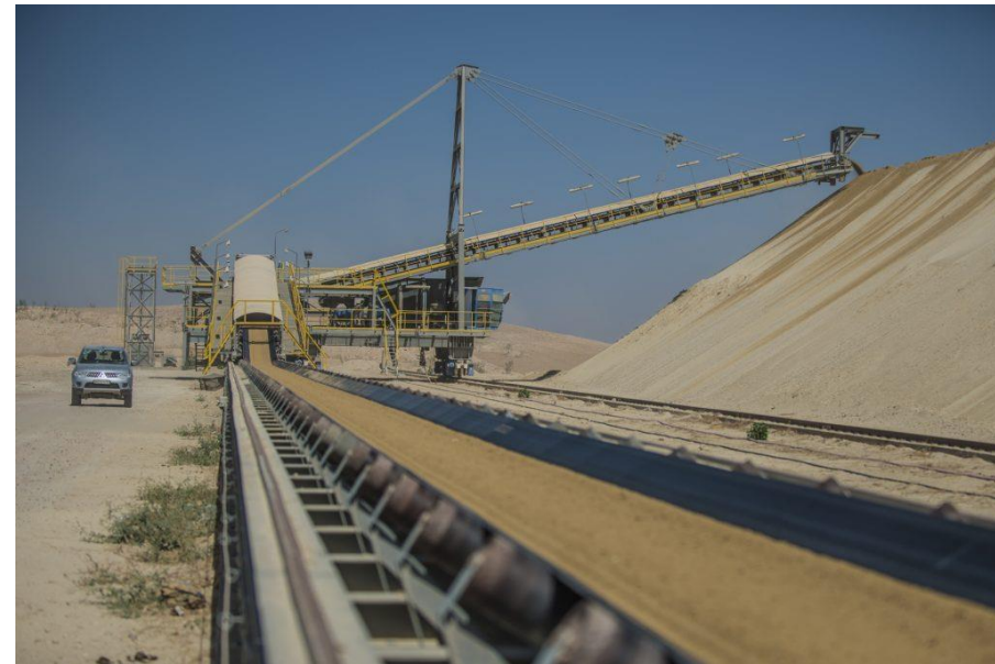
Benguerir Phosphate Mine
