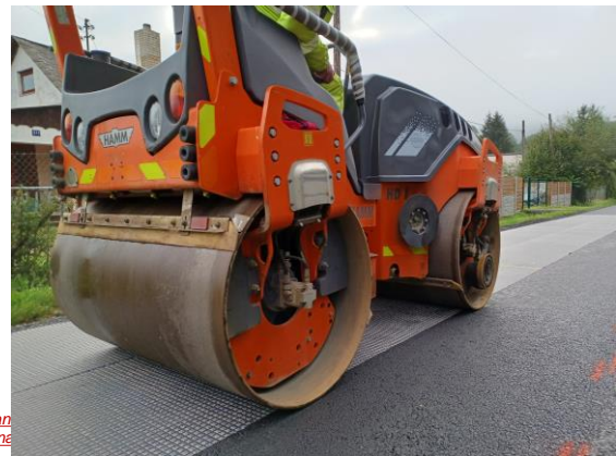
Pressure of reinforcement
