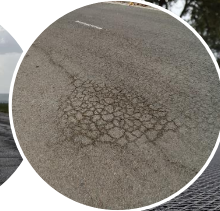
Example of cracking for area-wide repair
