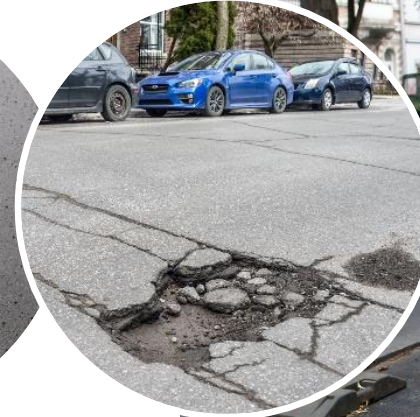
Example of cracking for local repair
