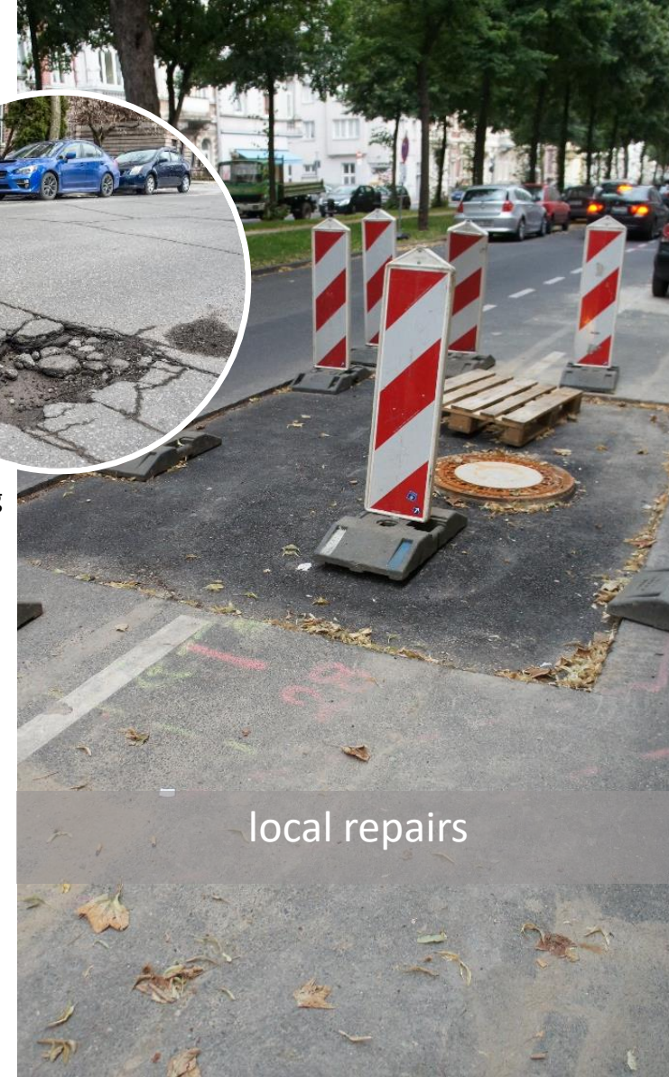
Example of cracking for local repair
