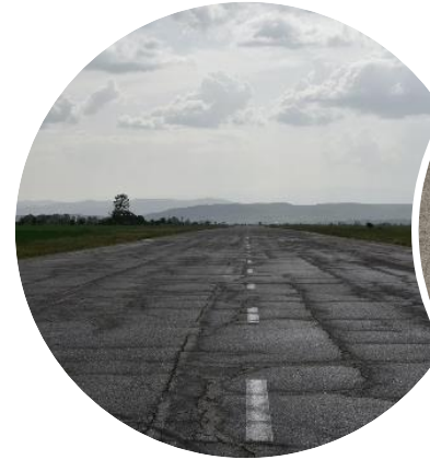
Example of cracking for area-wide repair
