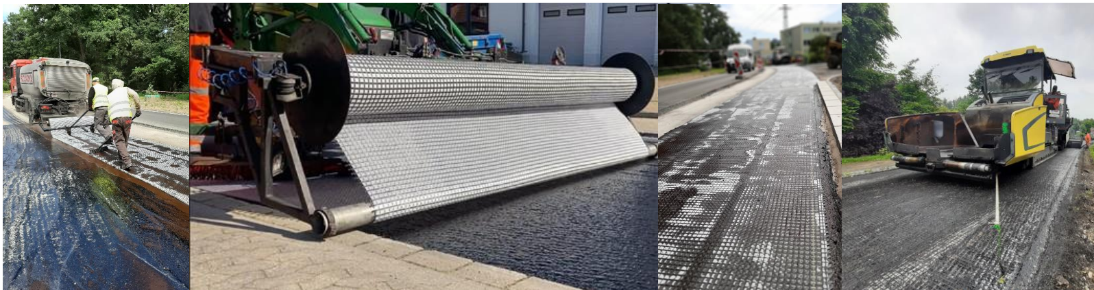
Application of GlasGrid CG/CGL on flat surface and pressure to fresh tack coat
