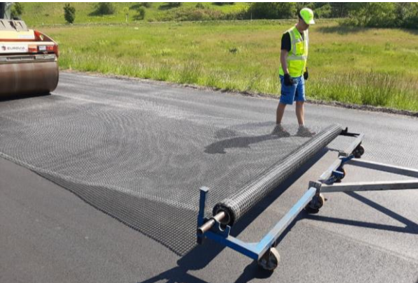
Application of GlasGrid GG on flat surface
