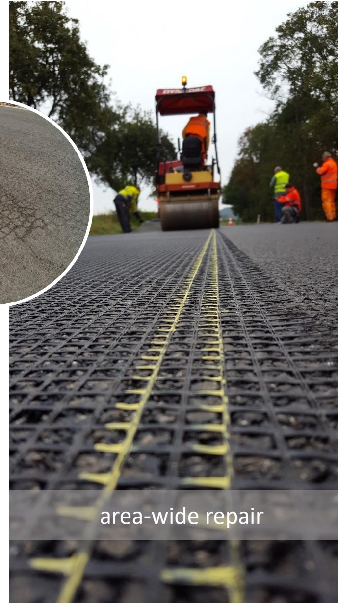
Example of cracking for area-wide repair
