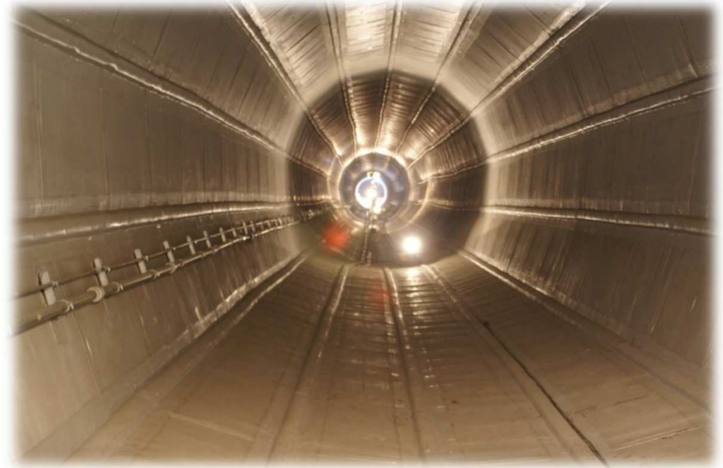
Belden Tunnel (near Albany) New York state United States
