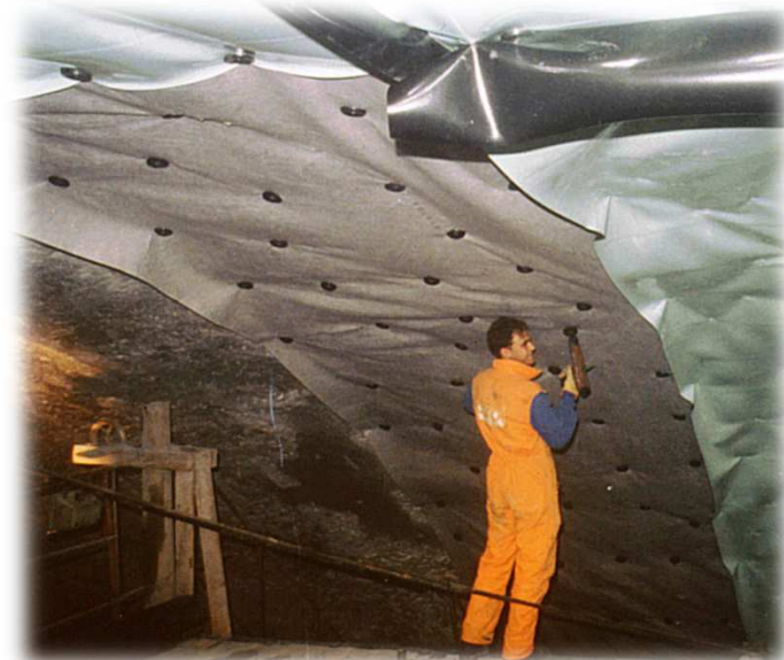
Driskos Tunnel – Greece
