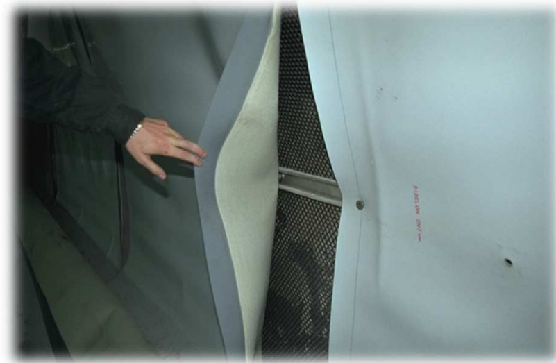
Spalov Tunnel - Czech Republic
