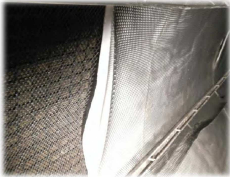
Chojlla Tunnel – Bolivia
