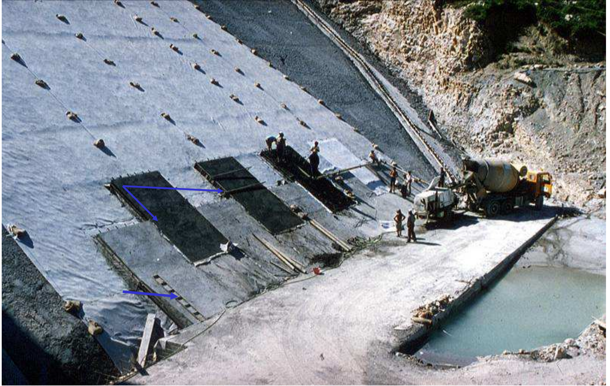
Casting of unreinforced concrete slabs, by alternate method
