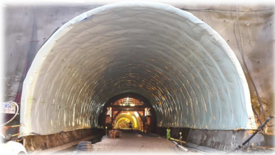
Tunnel of Marão - Portugal
