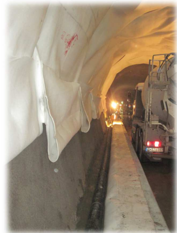
Gleitalm Tunnel – Austria
