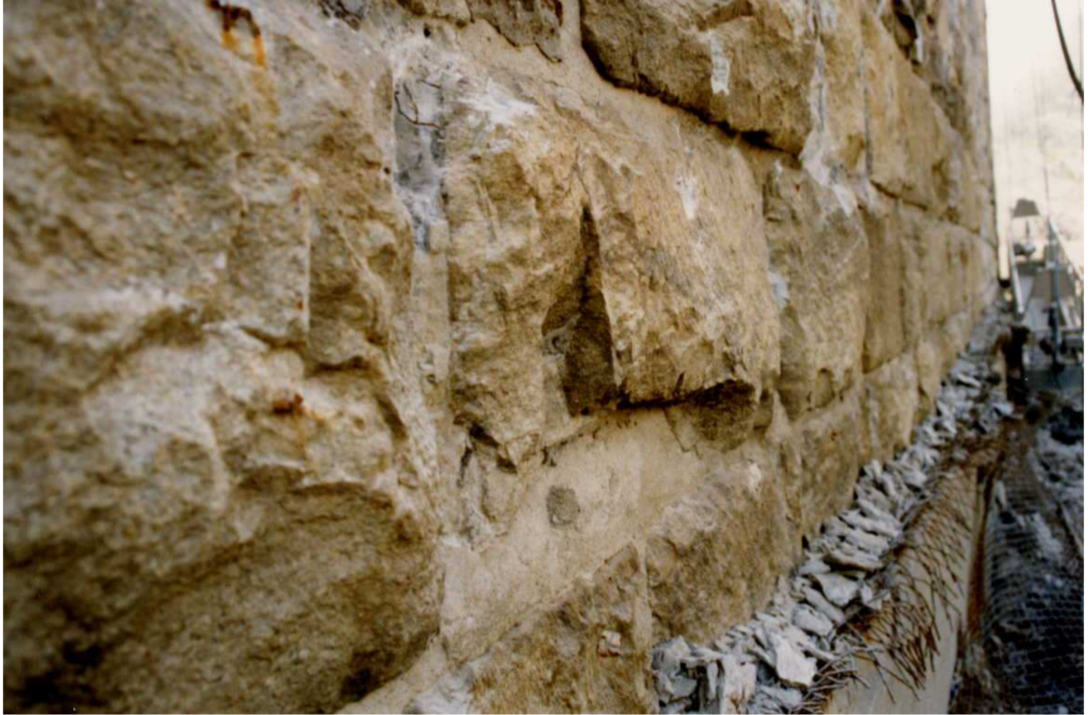
Dam masonry surface on which installation of composite geomembrane was required
